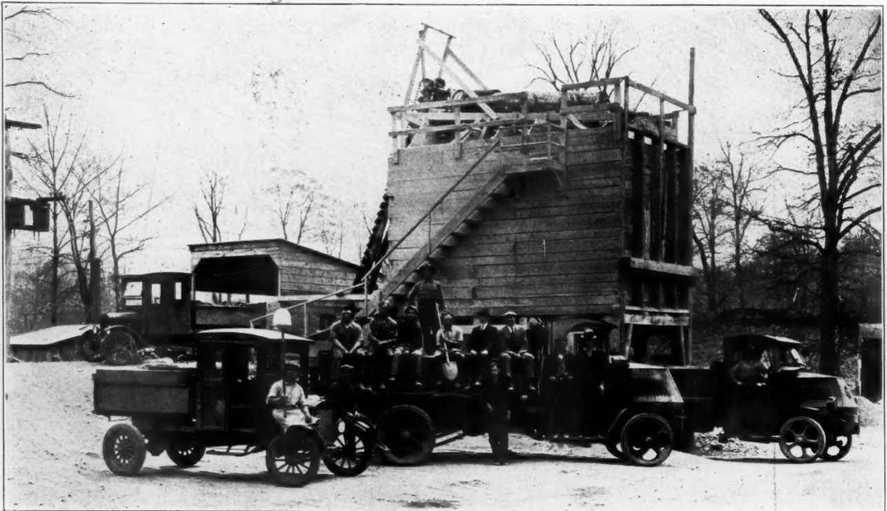
The Entire Force with the Crushing Plant in the Rear
